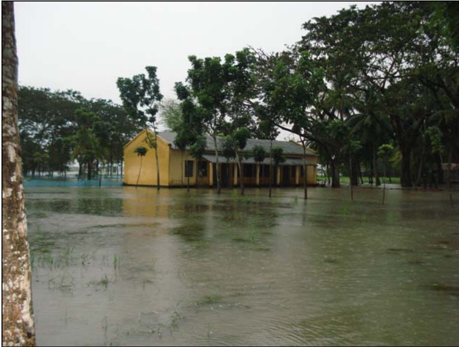
A School Building Inundated
