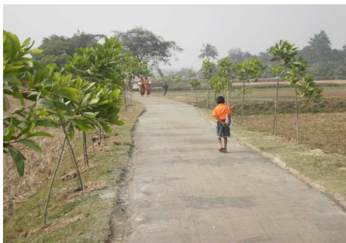
Concrete block road at Islampur, Sadar Upazila. Photo: SCBRMP
