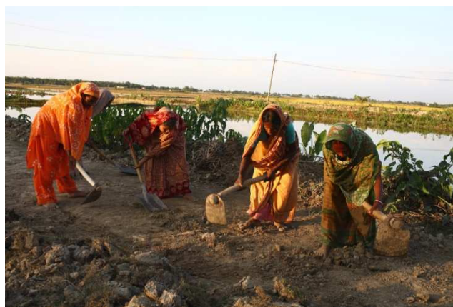
Women LCS members constructing road. Photo: Akash
