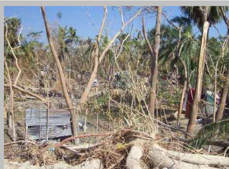
Damage caused by Sidr Photo: Fazlul Kader, FEDEC, PKSF
